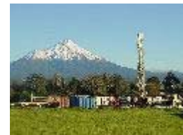
Drilling the Cheal 1 well, onshore Taranaki Basin, New Zealand.
